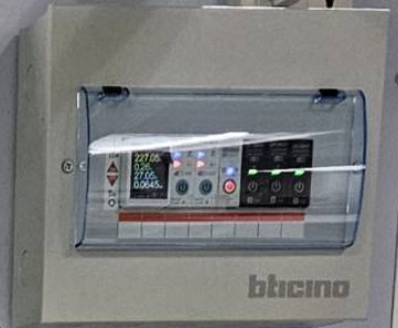
Smart Breaker 1P x 6 Ch + 2P x 1 KWS-302WF + TXCB2-VAP
